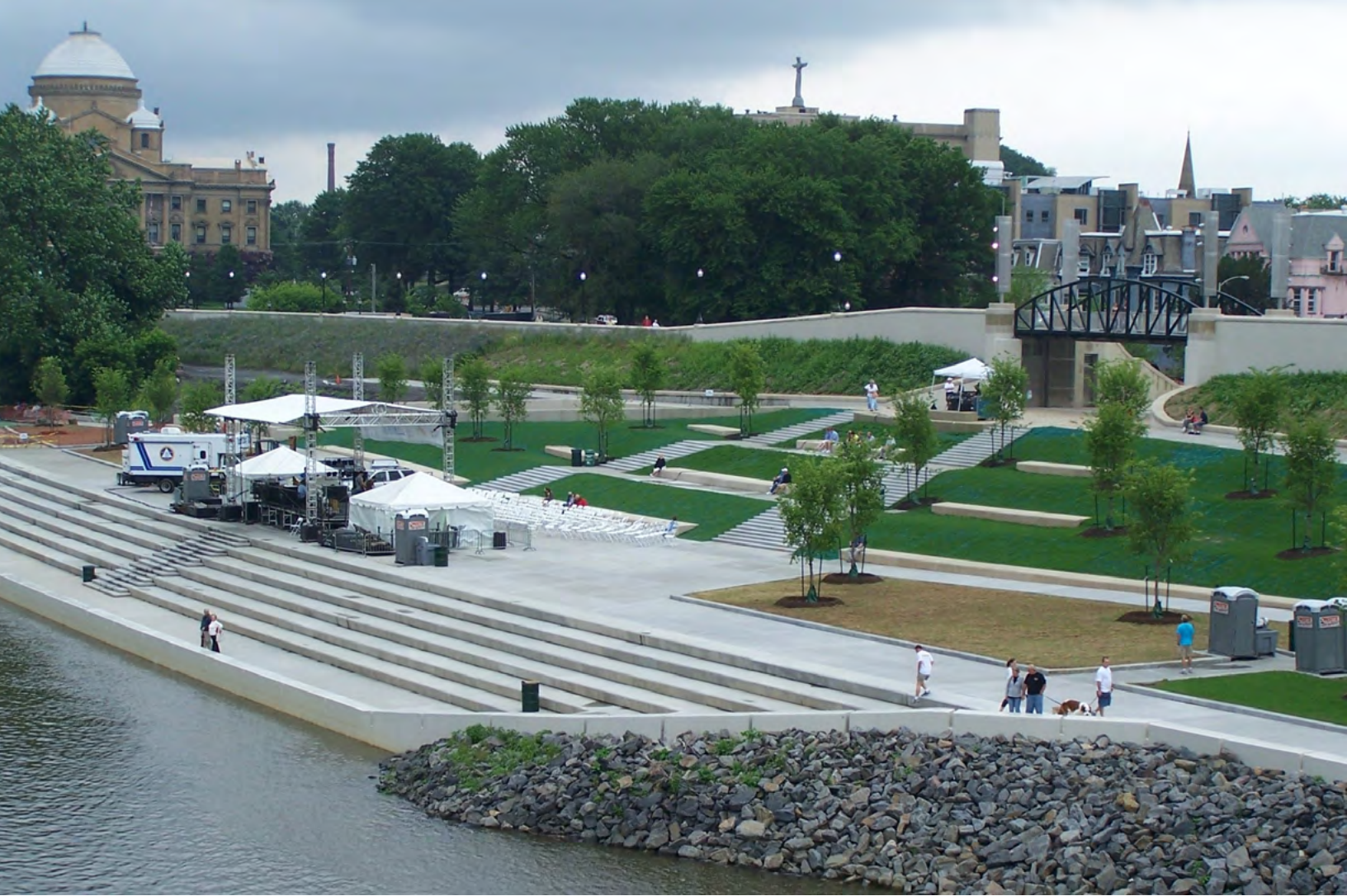
The Wyoming Valley Levee System, located in Wilkes-Barre, PA, June 2020
