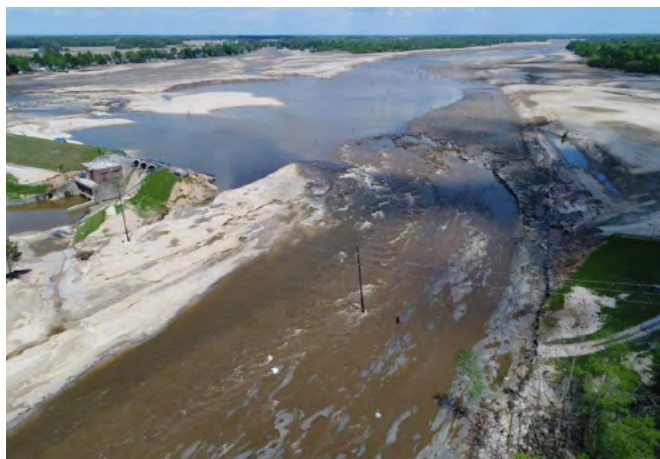
Edenville Dam After Failure on 5/19/2020, Looking Upstream
