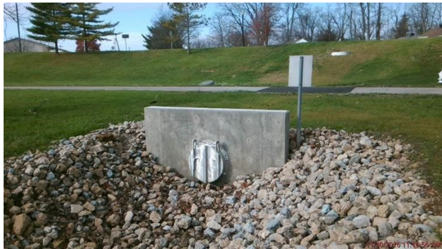
Figure 7-44: Example Headwalls with Flap Gates
