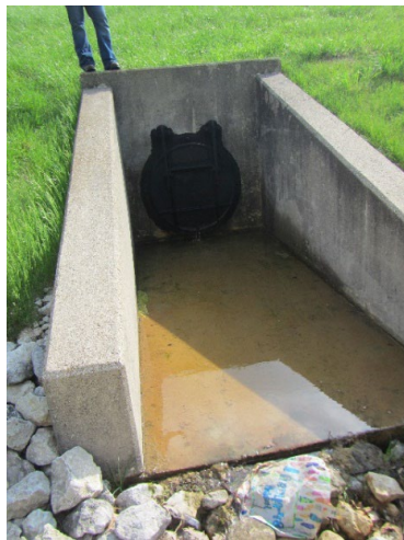
Figure 7-44: Example Headwalls with Flap Gates
