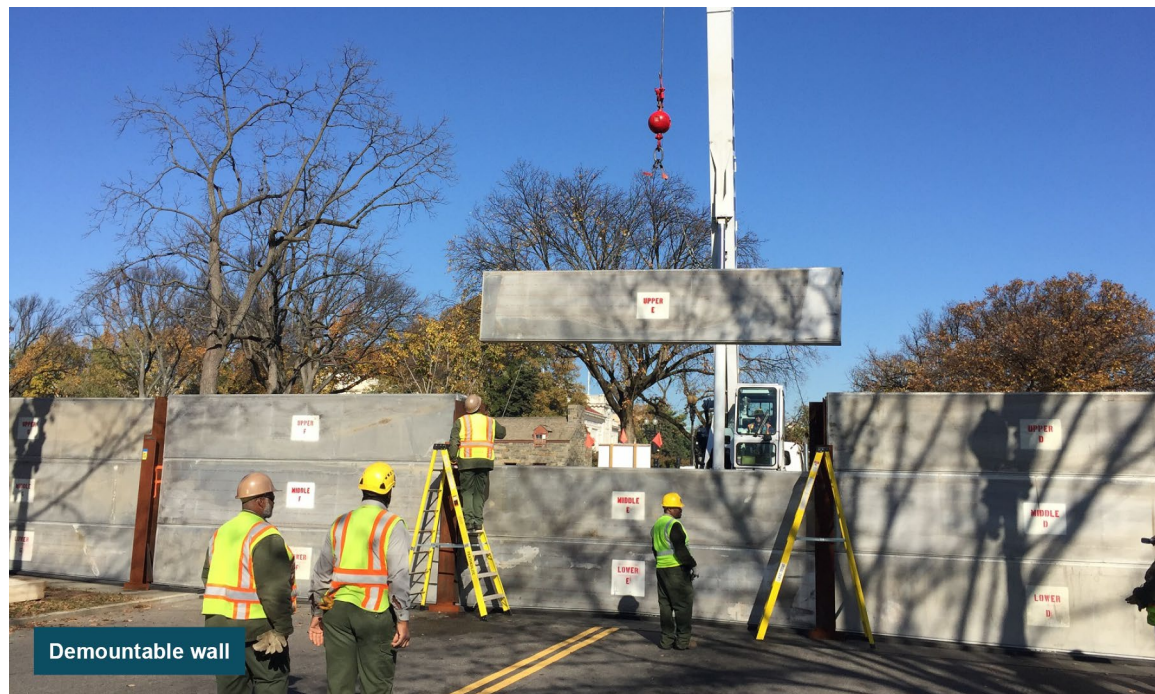
Figure 7-30: Example of Demountable Floodwall
