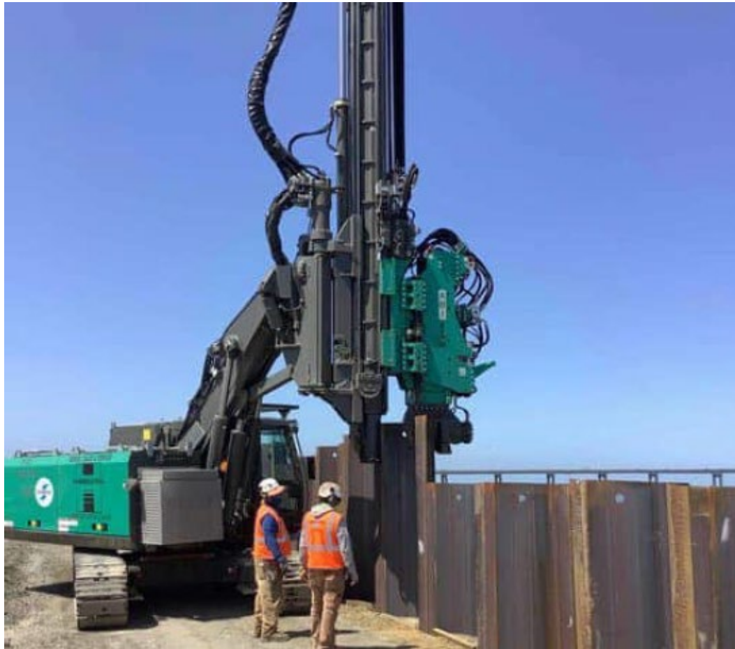
Figure 8-28: Example Pile Driving
