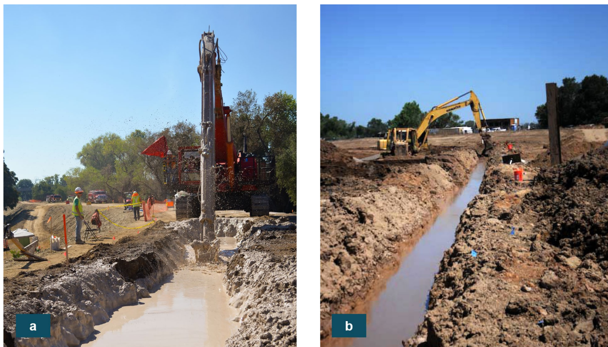
Figure 8-32: Example Open-Trench Cutoff Wall Construction
