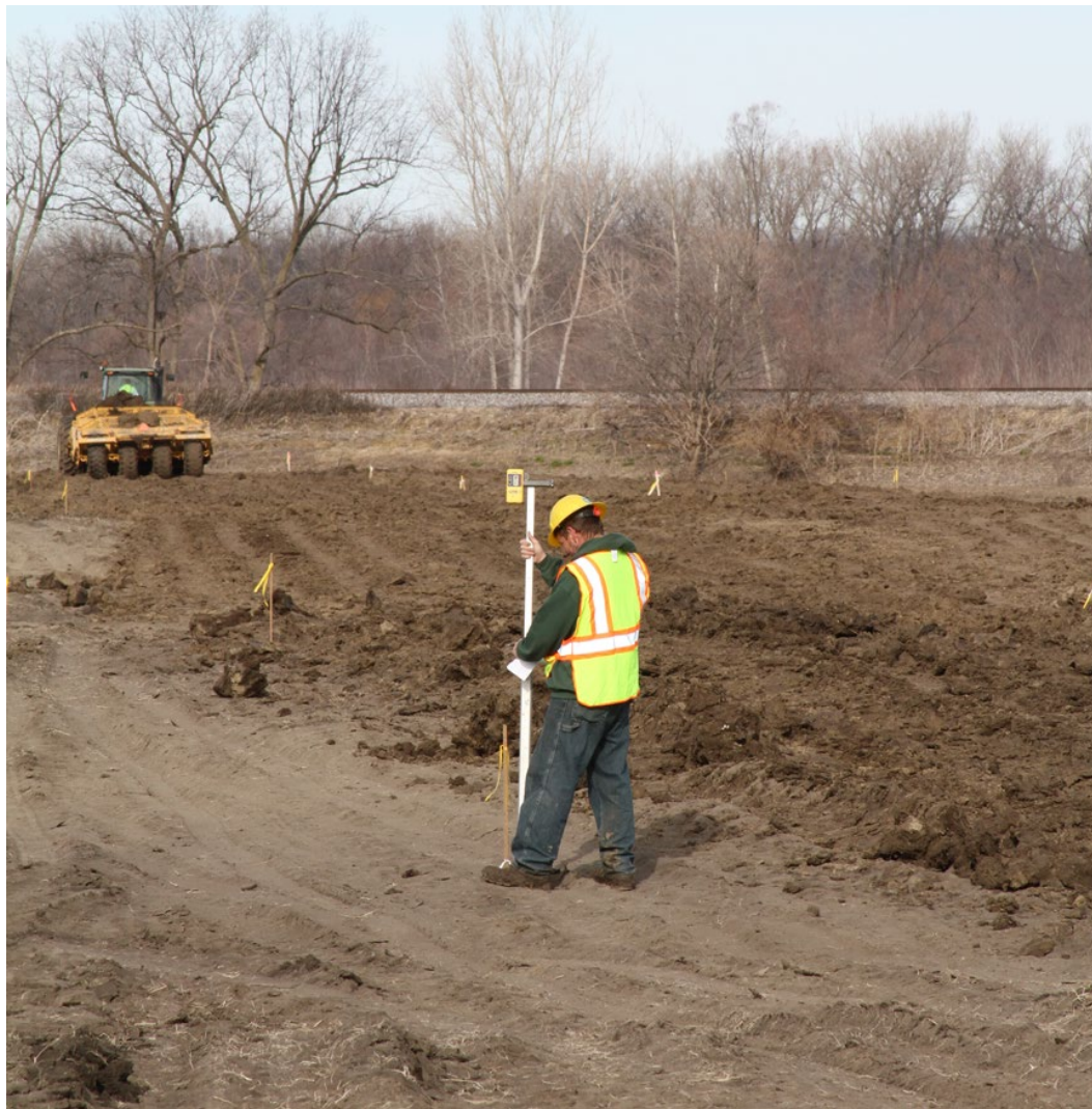
Figure 8-15: Example Survey Control
