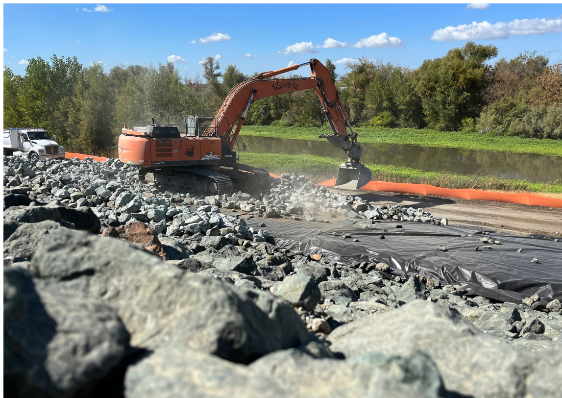
Figure 8-22: Example of Riprap Erosion Control Feature Construction
