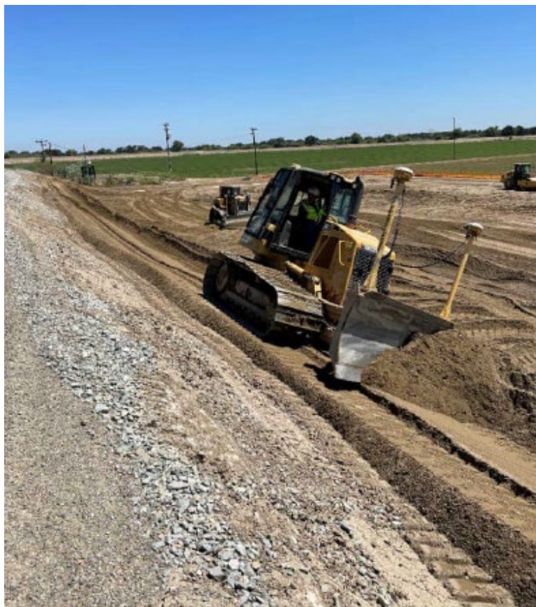
Figure 8-35: Example Construction of Landside Berm and Chimney Drain
