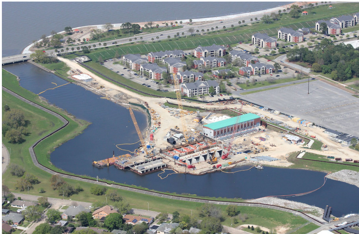
Figure 8-14: Example of Coastal Levee Construction
