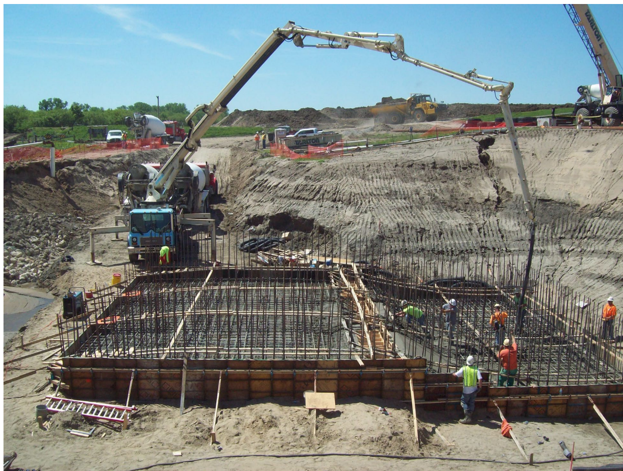
Figure 8-41: Example Construction of a Pump Station
