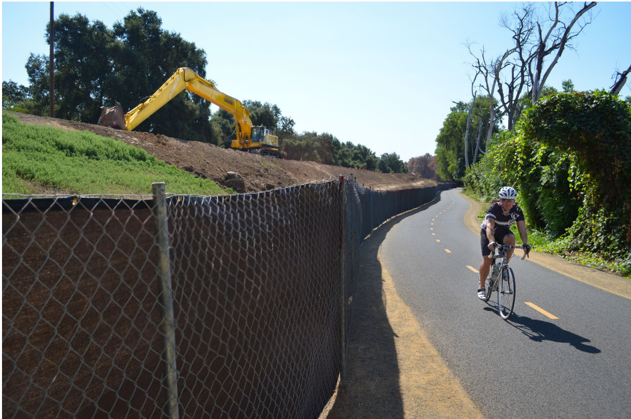
Figure 8-12: Example of Public Safety During Levee Construction
