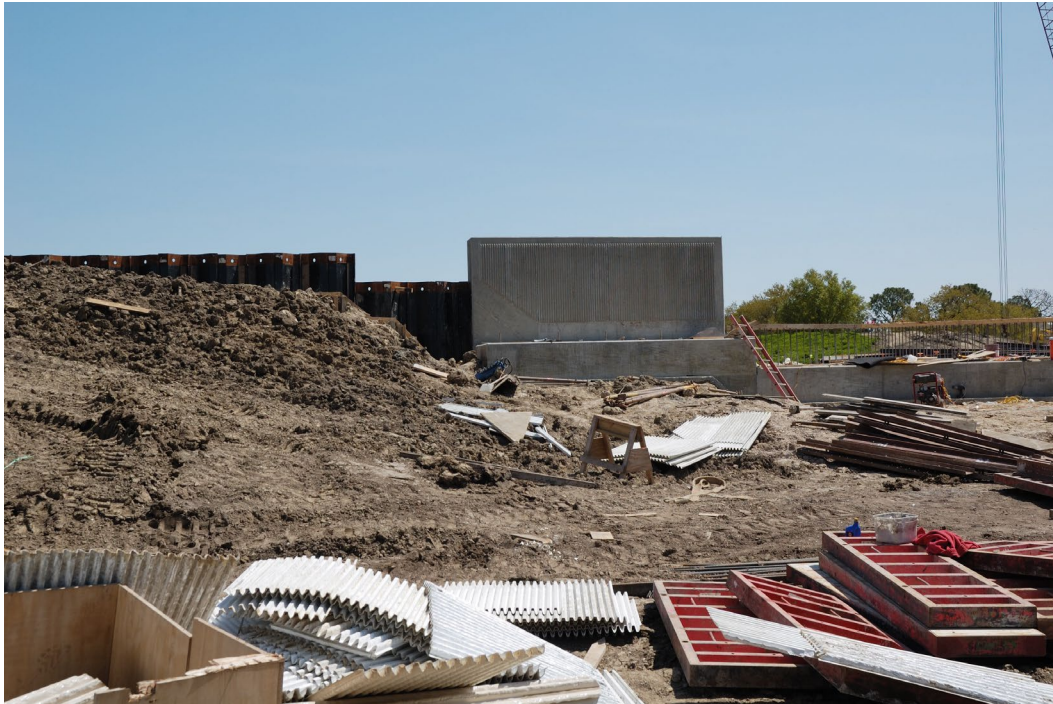
T-wall to I-wall to embankment transition under construction in New Orleans, Louisiana.
