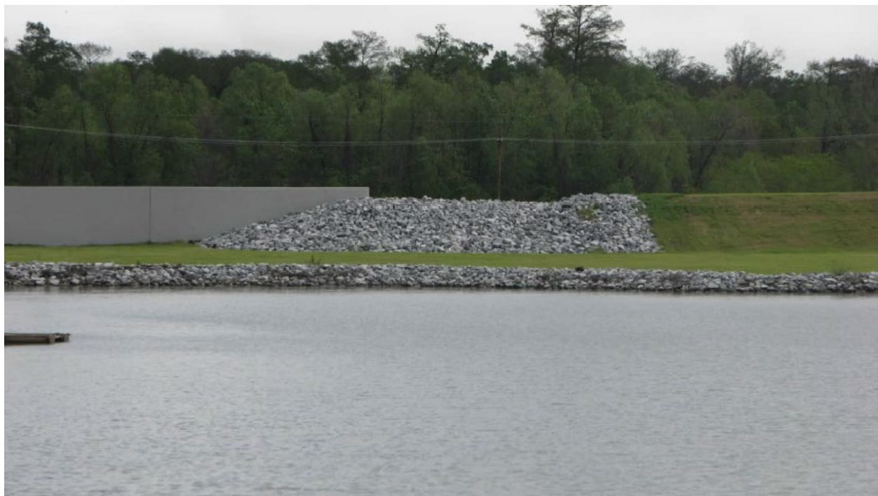
Figure 8-31: Example Levee Transition Connection (Embankment and Floodwall)
