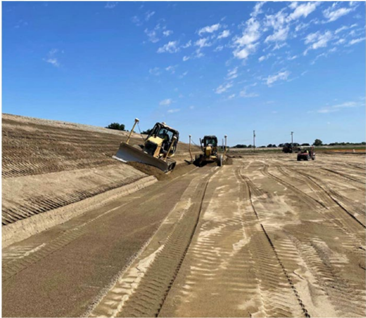
Figure 8-21: Example Embankment Slopes
