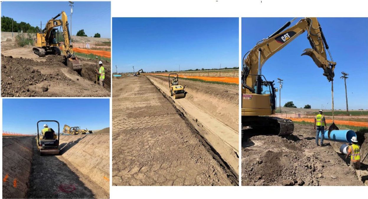
Figure 8-39: Example of Landside Interior Drainage Construction
