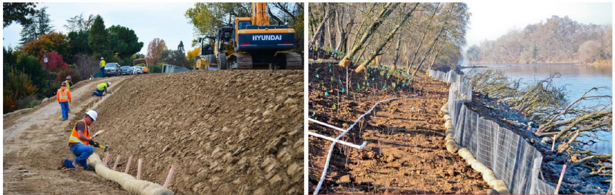
Figure 8-13: Example of Temporary Erosion Protection
