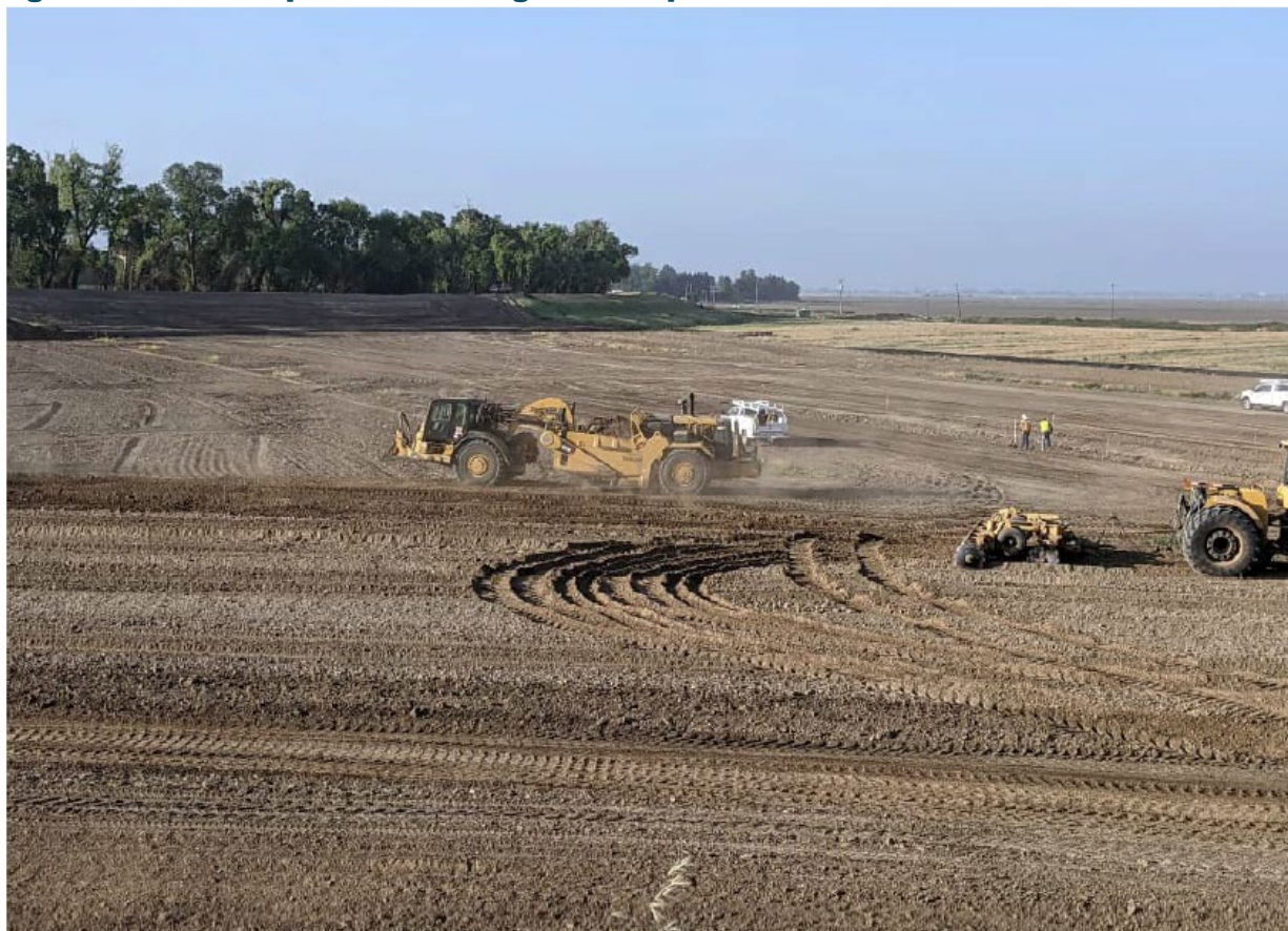
Figure 8-16: Example Levee Subgrade Preparation
