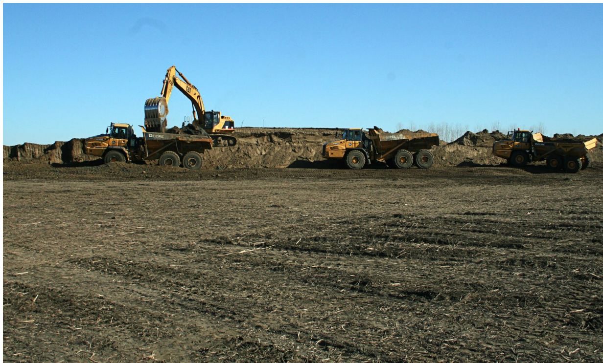
Figure 8-18: Example Borrow Source Excavation
