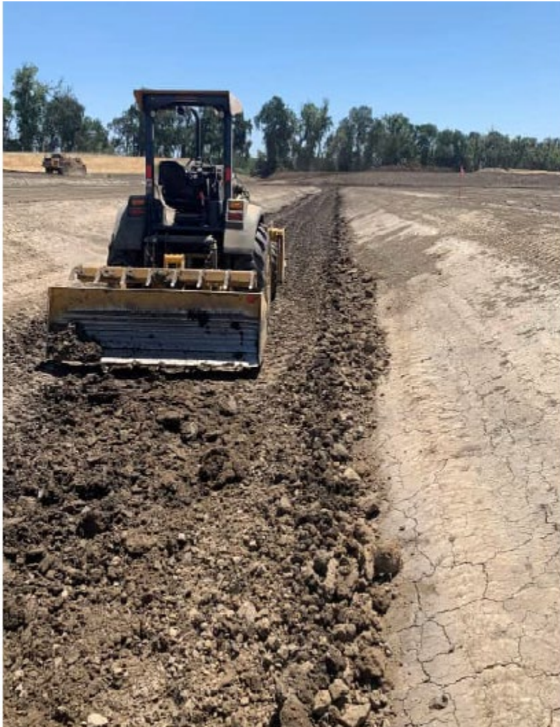
Figure 8-17: Example Inspection Trench
