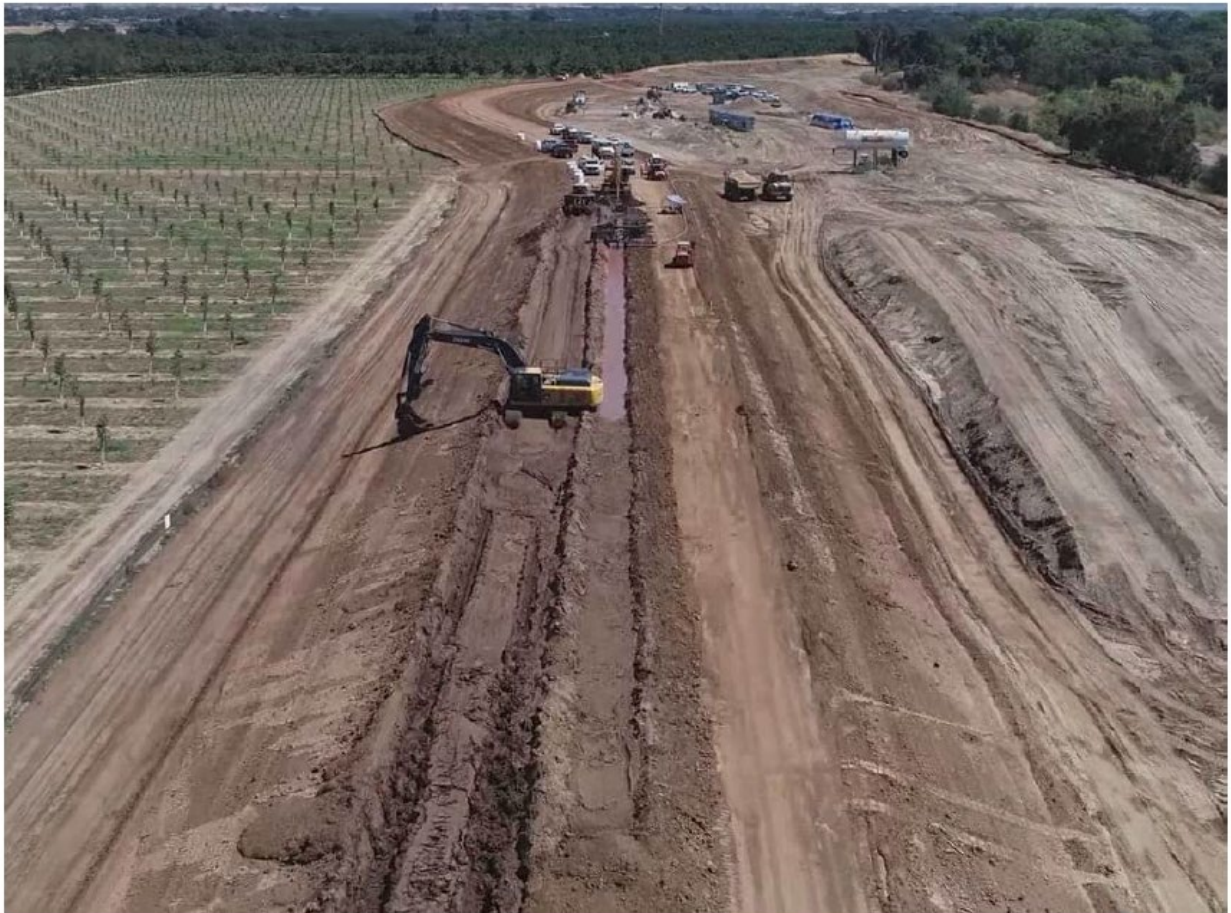
Figure 8-10: Aerial View of Levee Construction
