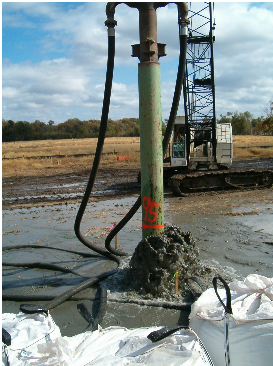
Figure 8-38: Example Relief Well Construction
