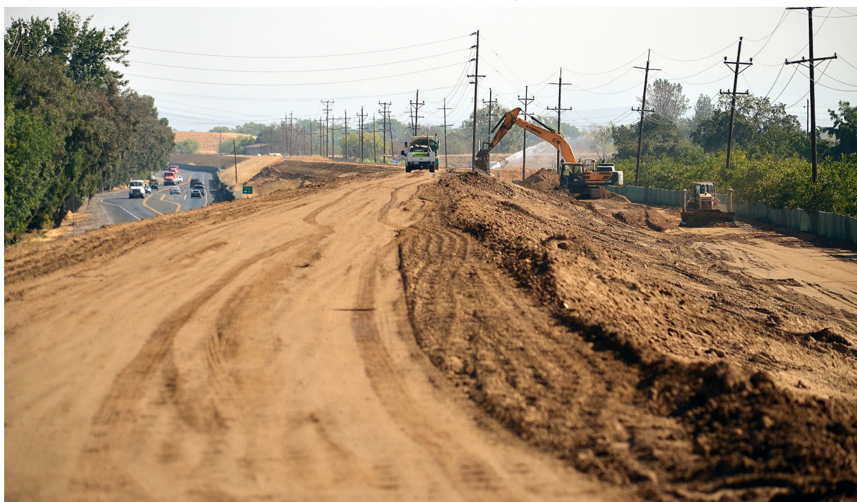
Figure 8-4: Example of a Levee Construction Project
