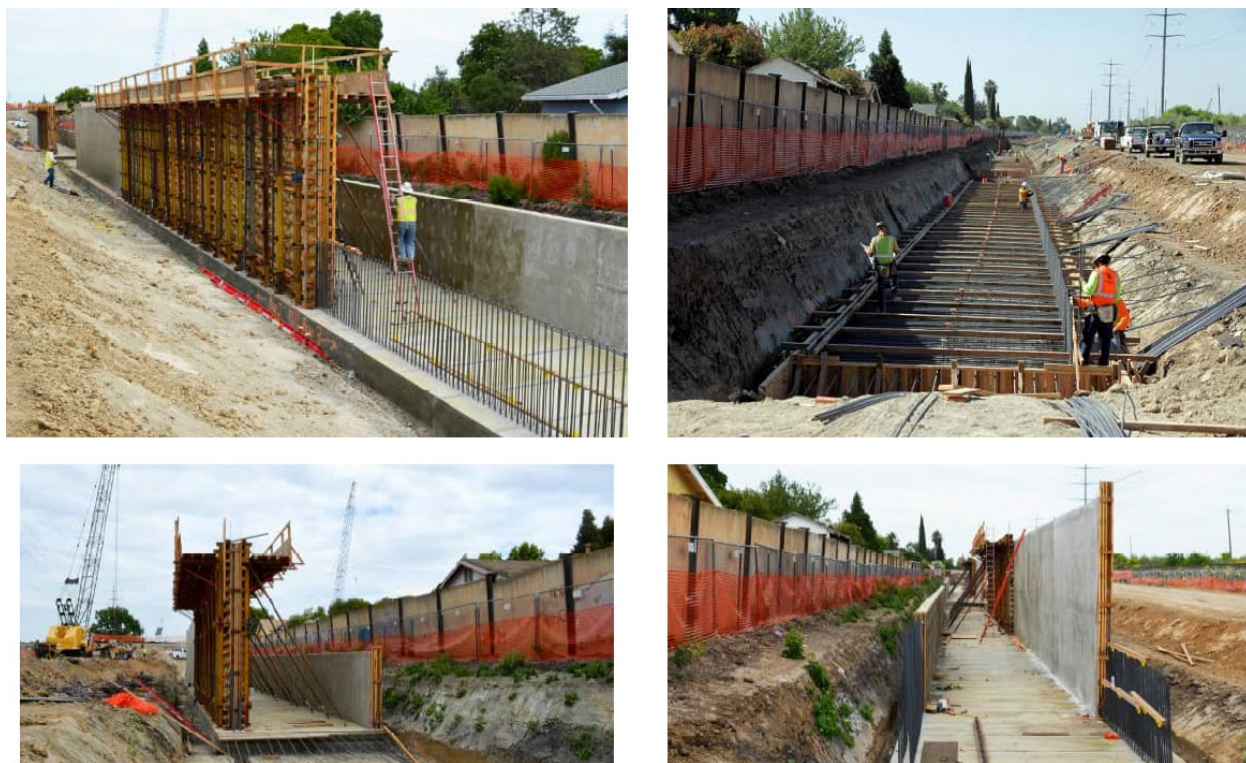
Figure 8-26: Example Floodwall Foundation Construction
