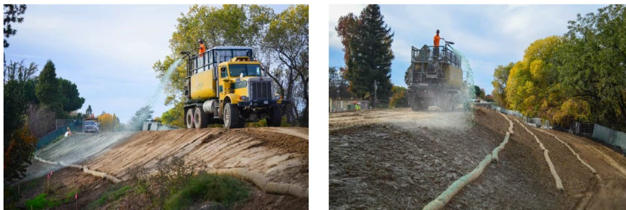
Figure 8-23: Example of Hydroseeding for Erosion Control
