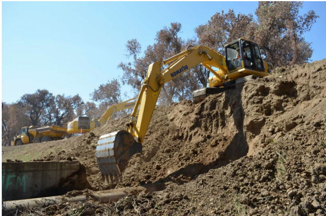
Figure 8-25: Example of Excavation of an Abandoned Utility
