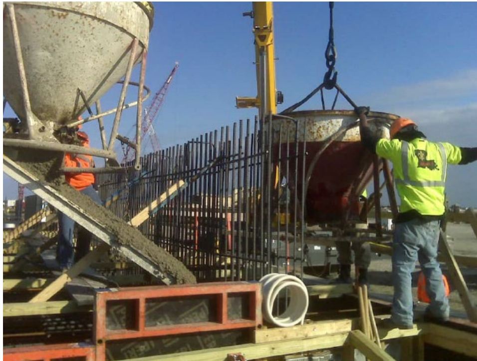
Figure 8-27: Example Concrete Placement for Floodwalls
