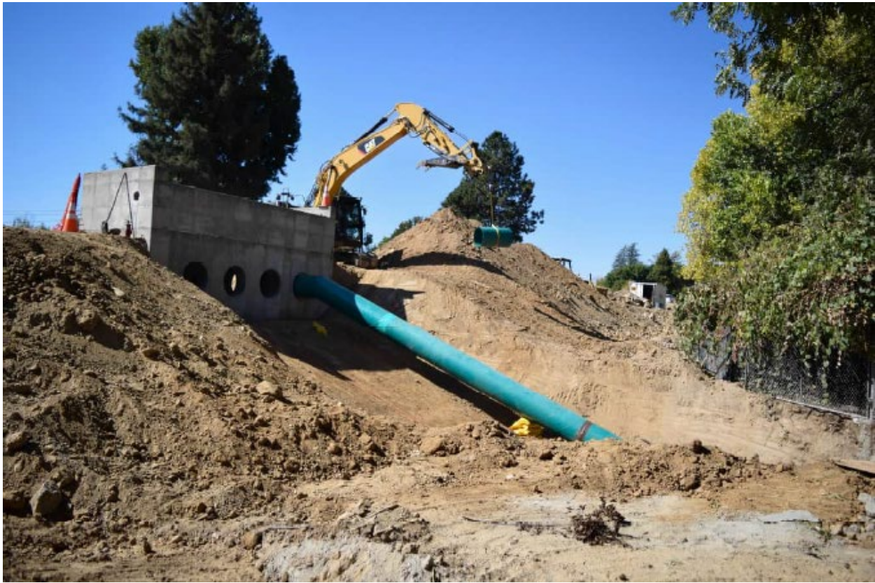
Figure 8-40: Example Interior Drainage Pump Station
