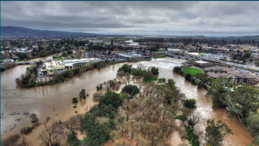
The photo displays the elevated railroad and roadway bridges over the new bypass channel. The bypass channel converges with the more natural river downstream (Napa County Flood Control & Water Conservaton District, 2023).
