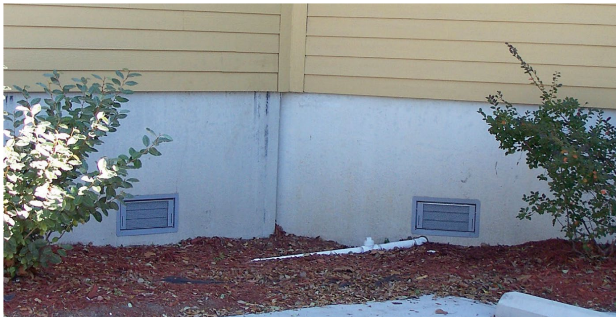
Figure 12-10: Wet Floodproofed Building with Flood Openings
