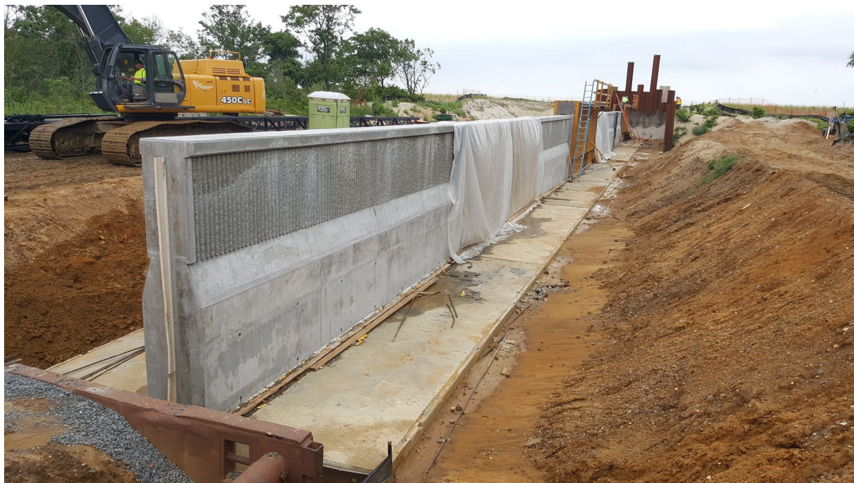
Figure 8-9: Levee Construction Performed by a Constructor
