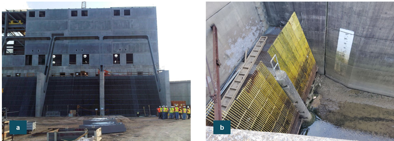
Figure 9-37: Examples of Pump Station Trash Racks
