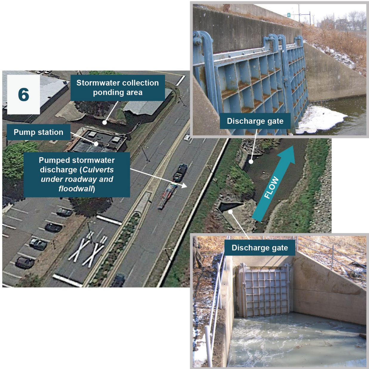
Figure 2-61: Example of Interior Drainage System
