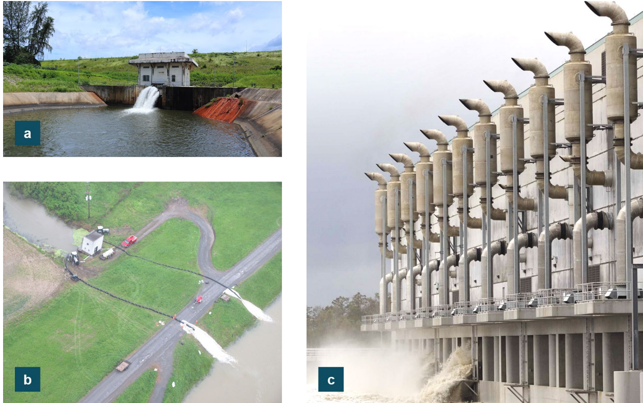
Figure 9-36: Examples of Pump Station Scale and Conditions
