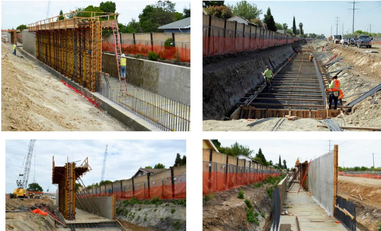
Figure 8-26: Example Floodwall Foundation Construction
