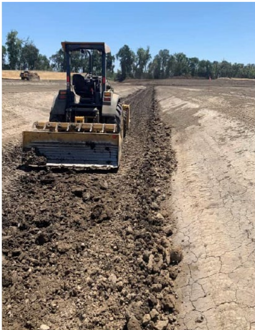
Figure 8-17: Example Inspection Trench
