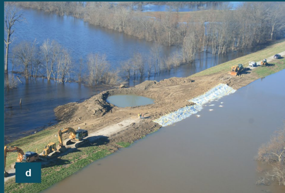
(a) Sinkhole caused by a buried pipe failure. (b and c) In 2013, emergency levee repairs occurred at a pipe failure along the Mississippi River. (d) A second pipe failure occurred a few years later at the same Mississippi River site.
