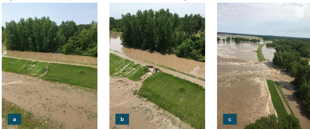
Figure 9-19: Example of Animal Burrows Leading to Levee Breach
