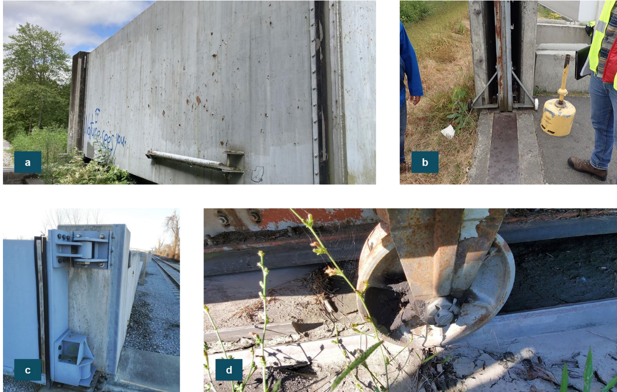
Figure 9-23: Examples of Movable Gate Inspection Observations
