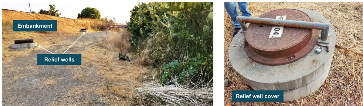
Figure 2-40: Example Relief Well
