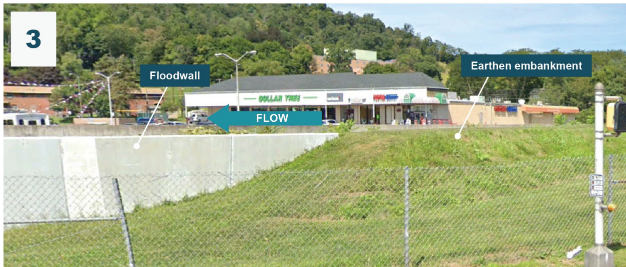
Figure 2-58: Example of Embankment Tie-in to Floodwall
