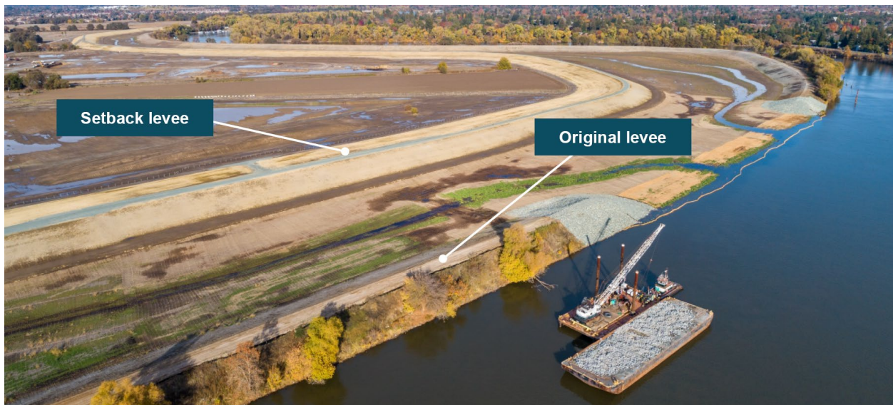
Figure 2-7: Example Setback Levee
