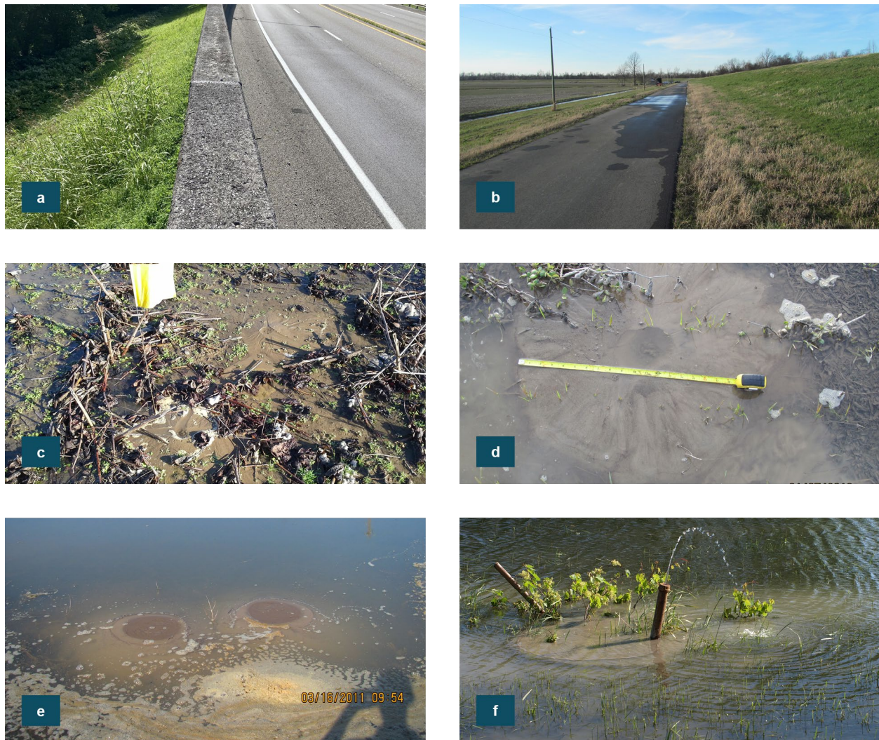
(a) Isolated vegetation is denser and taller than the nearby vicinity as an indication of potential seepage. (b) Throughseepage emerging at the landside toe of a levee on the Mississippi River during a flood. (c) Very small sand boils (pin boils) moving negligible amounts of soil near the toe of a Mississippi River levee. (d) Medium sand boil transporting material along the Mississippi River levee. (e) Two large sand boils in a pump station ponding area in Illinois. Note the 'milkshake foam' in the foreground is often an indicator that sand boils are forming underwater. (f) Material emerging from around a deteriorated piezometer during a flood near the conflux of the Ohio and Mississippi Rivers. This can be a particularly concerning situation since the damaged piezometer can provide a direct pathway for seepage.
