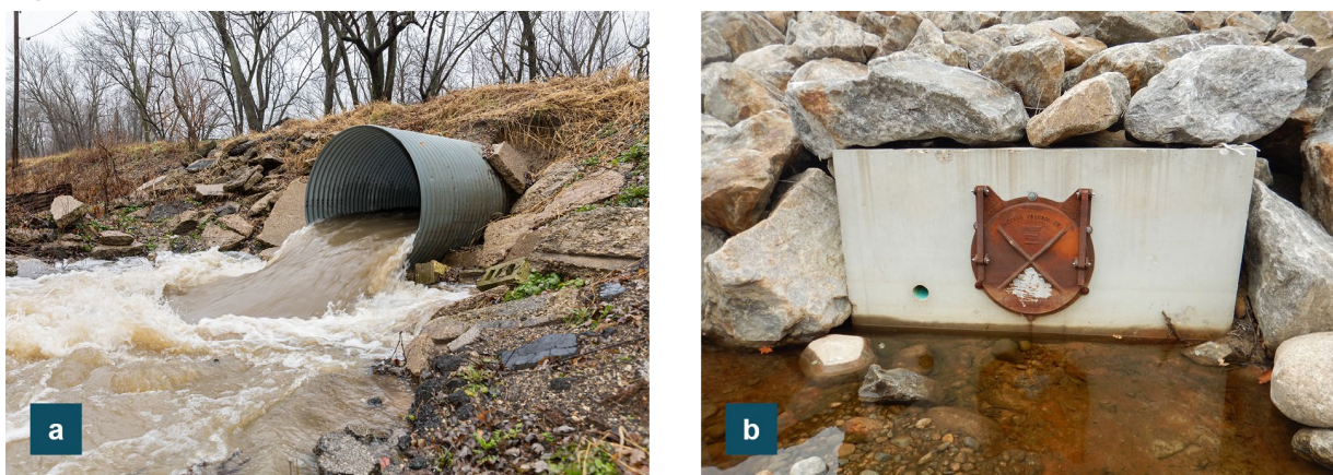
Figure 9-30: Concrete Headwall Conditions
