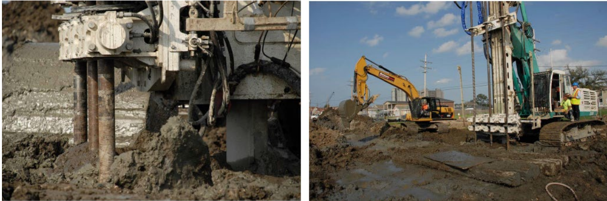
Figure 8-33: Example Mix-in-Place Cutoff Wall Construction
