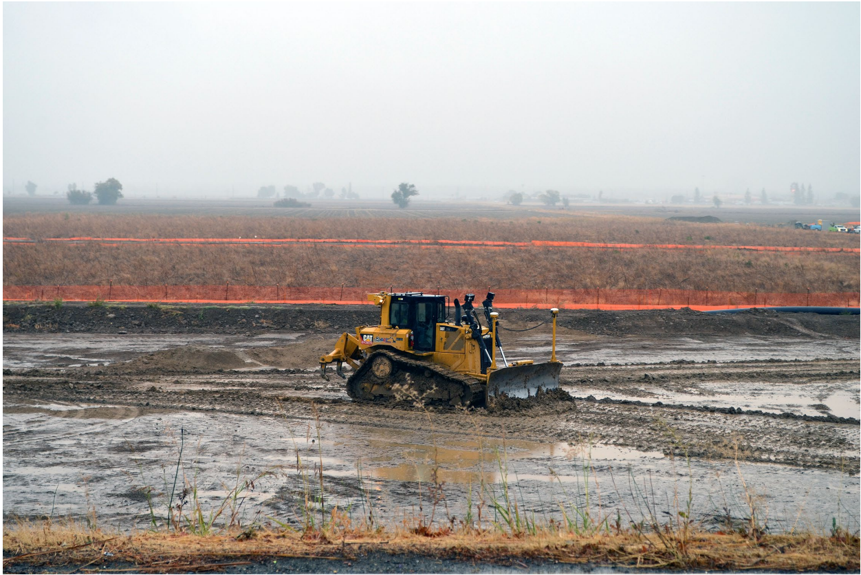
Figure 8-8: Inclement Weather Impacting Levee Construction
