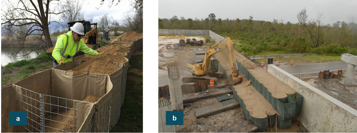
Figure 2-32: Example Soil/Gravel Basket Closures
