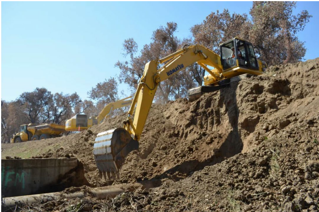
Figure 8-25: Example of Excavation of an Abandoned Utility
