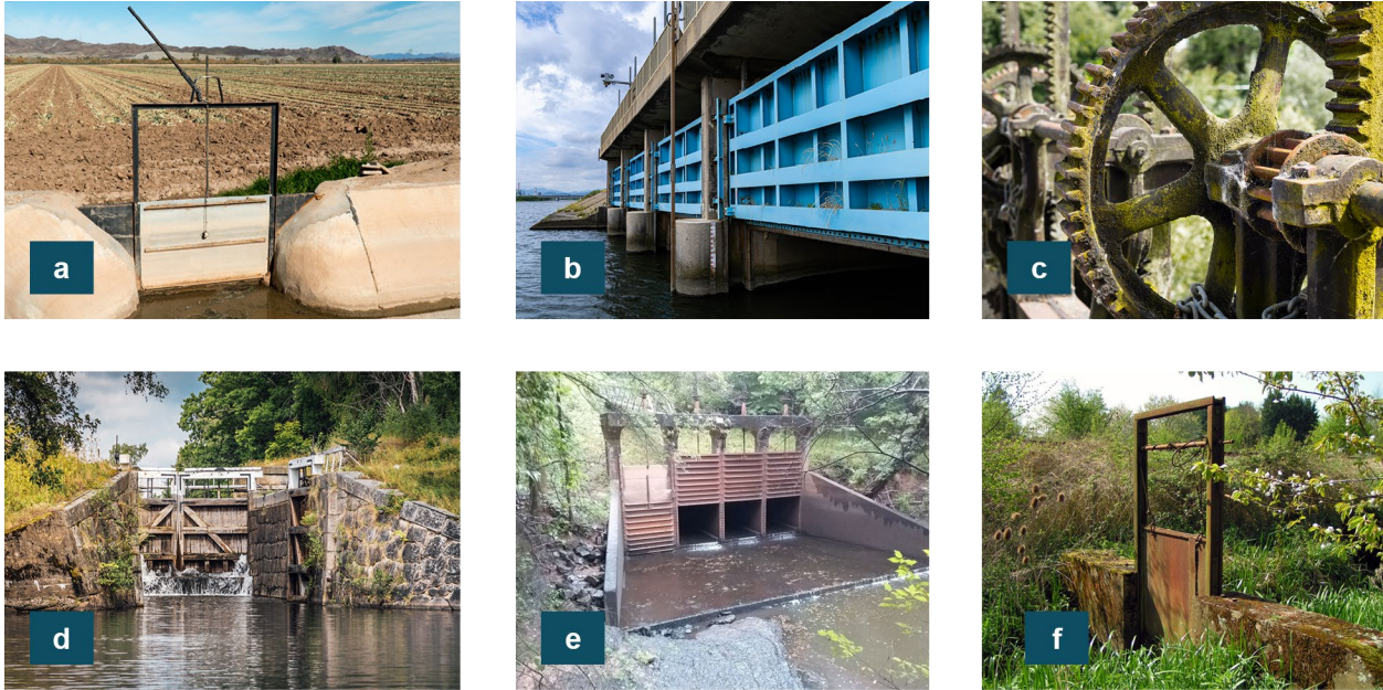
Figure 9-31: Examples of Sluice Gate Scale and Conditions
