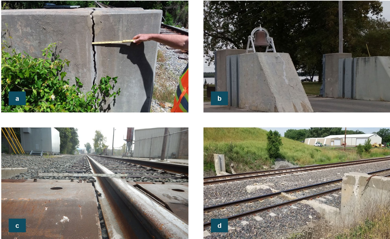
Figure 9-24: Examples of Structural Assembled Closure Inspection Observations
