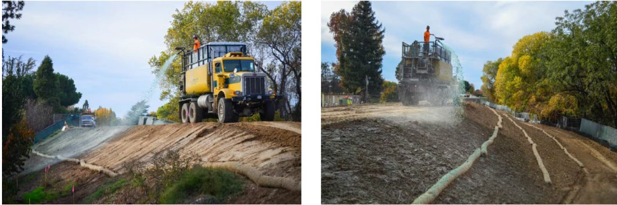
Figure 8-23: Example of Hydroseeding for Erosion Control
