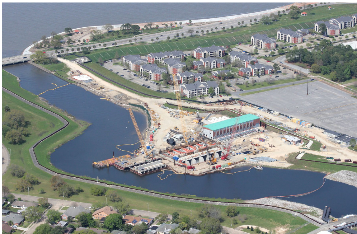
Figure 8-14: Example of Coastal Levee Construction
