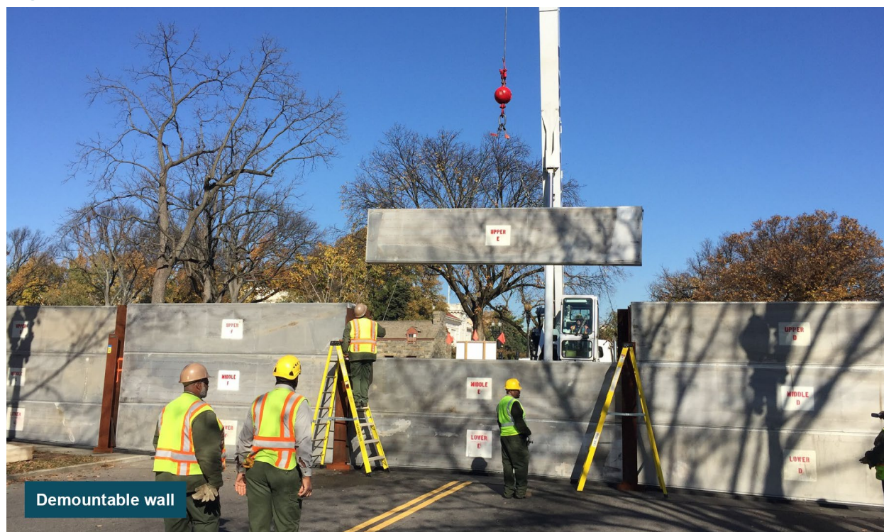
Figure 2-19: Example Demountable Walls
