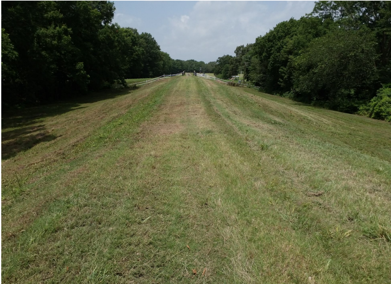
Figure 9-14: Example of Localized Crown Settlement
