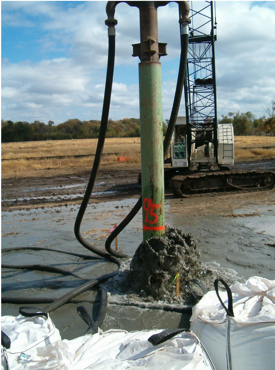
Figure 8-38: Example Relief Well Construction
