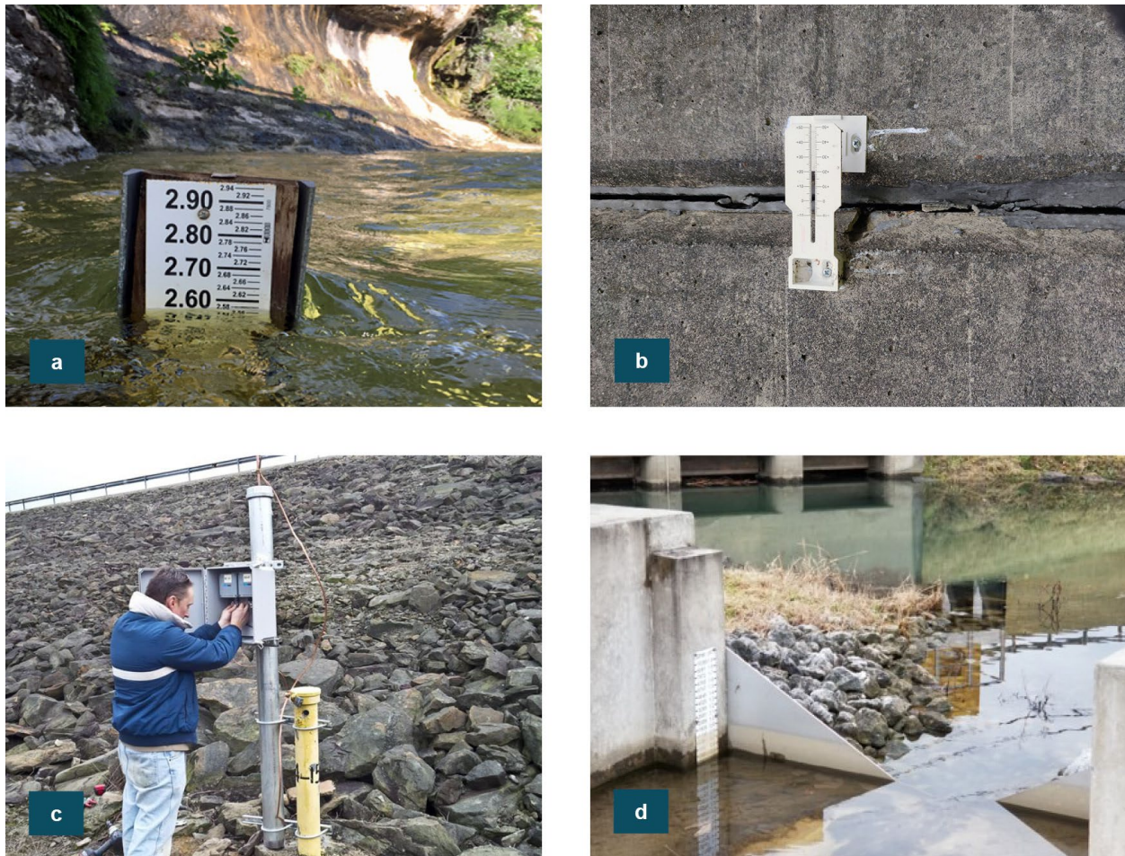
Figure 2-50: Typical Levee Instrumentation
