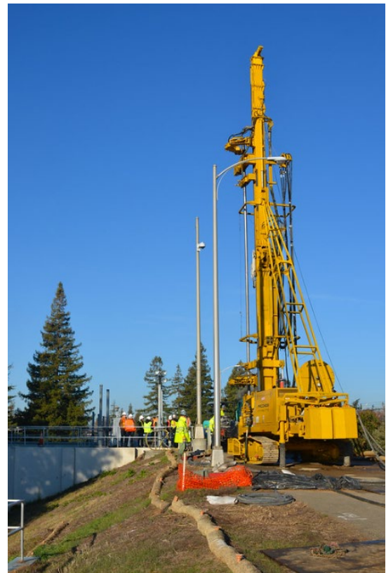
Geotechnical investigation may involve drilling borings to understand underlying geology.
