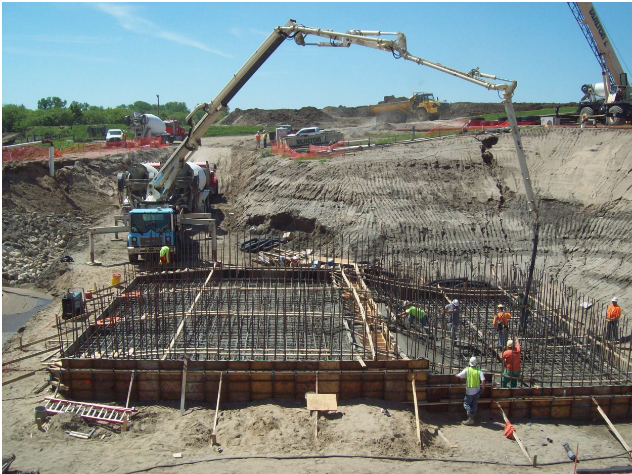
Figure 8-41: Example Construction of a Pump Station
