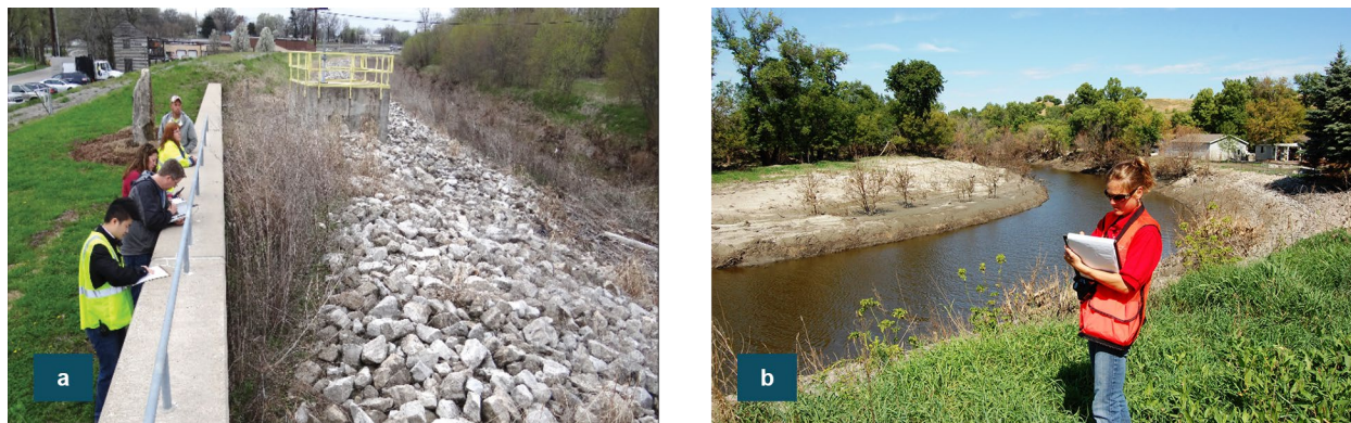
(a) Inspectors making notes during a floodwall inspection. (b) Inspector making notes during a levee inspection at the Souris River Levee in Ward County, North Dakota.
