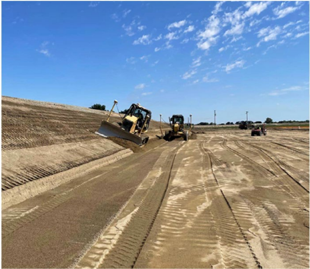
Figure 8-21: Example Embankment Slopes
