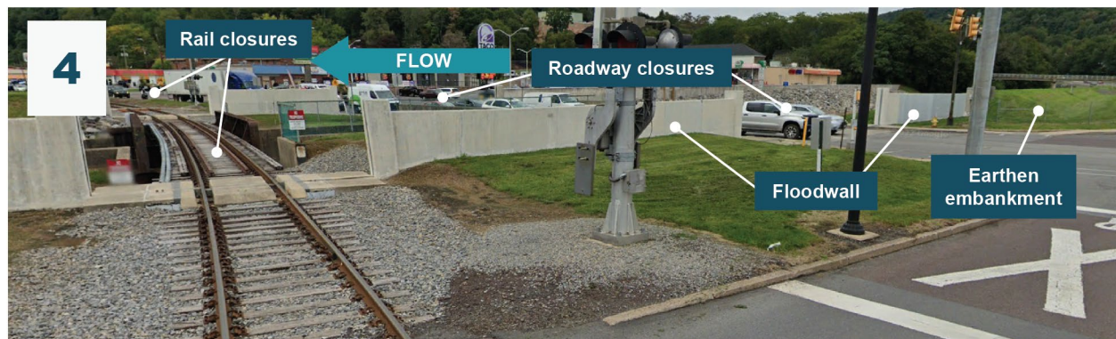
Figure 2-59: Example of Railway and Roadway Closures
