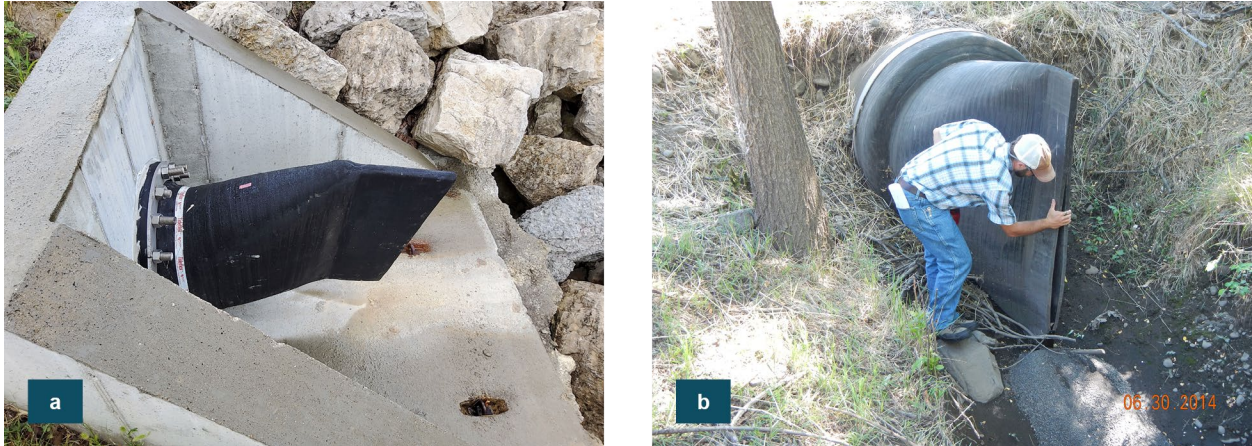
Figure 9-33: Examples of Duckbill Valve Scale and Condition
