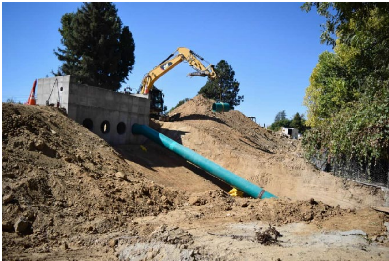
Figure 8-40: Example Interior Drainage Pump Station
