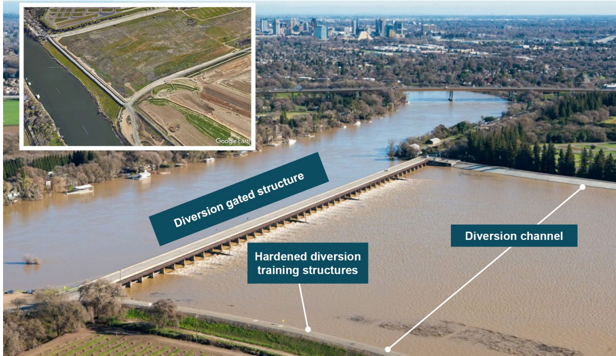
Figure 2-42: Typical Floodway Channel
