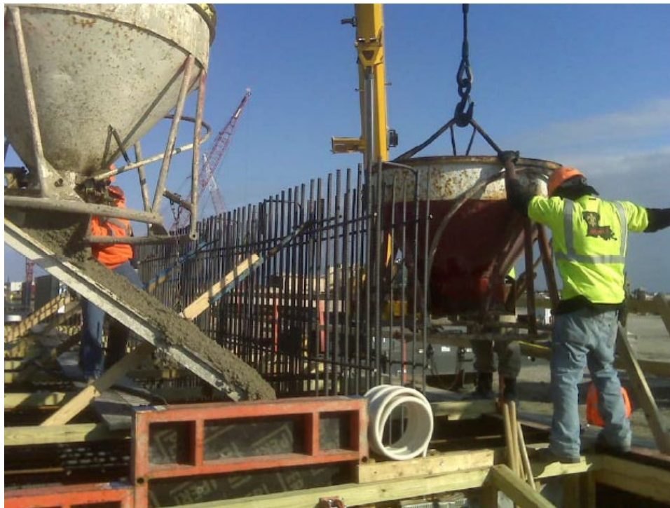
Figure 8-27: Example Concrete Placement for Floodwalls
