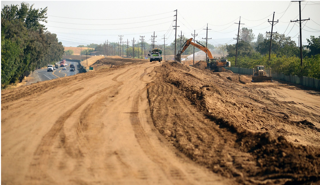
Figure 8-4: Example of a Levee Construction Project
