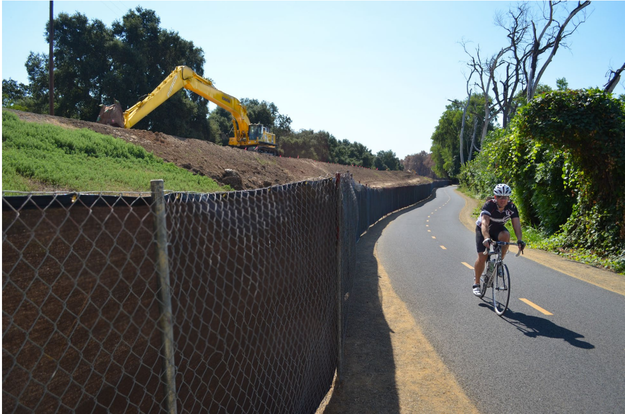
Figure 8-12: Example of Public Safety During Levee Construction
