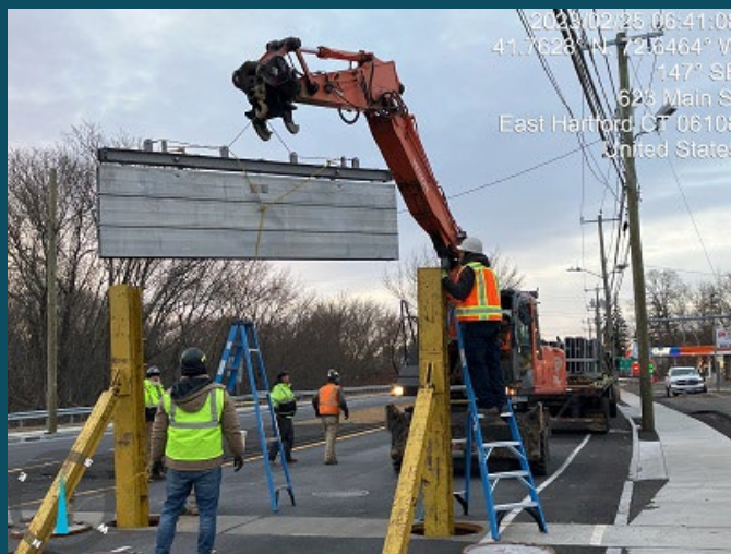
Annual exercise to practice stoplog closure installation in East Hartford, Connecticut.
