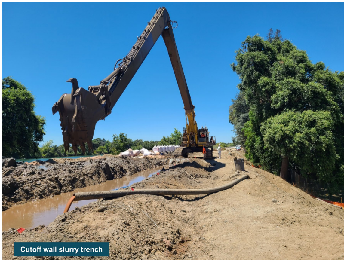
Figure 2-36: Cutoff Wall Under Construction
