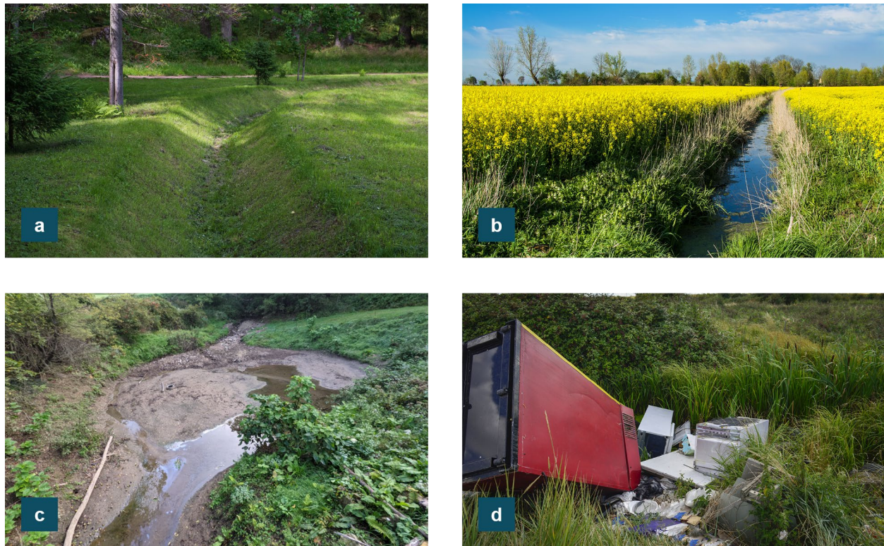
Figure 9-35: Examples of Drainage Ditch Conditions
