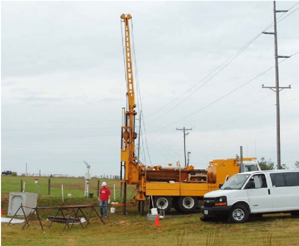
Figure 7-11: Example Field Investigations
