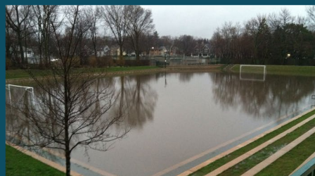
Washington Park in Downers Grove, Illinois before and after extreme rain. The park was designed to allow for storm water detention after rain events.
