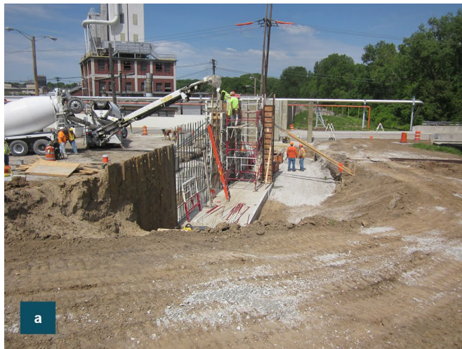
Figure 2-16: Examples of Floodwalls
