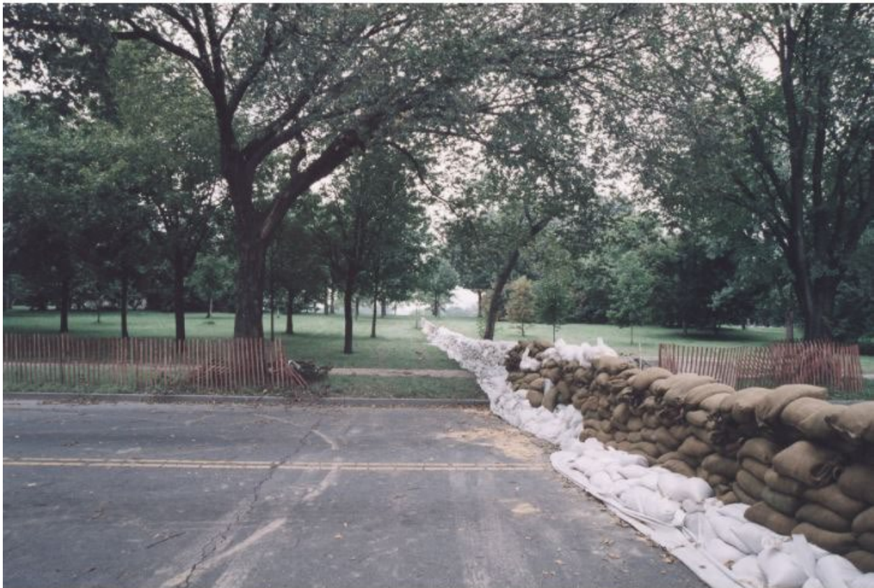
Levee closure across a roadway using sandbags in Washington, D.C.
