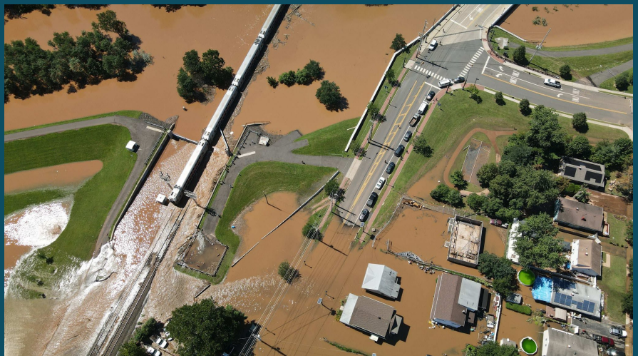
Aerial view of a train blocking operation of a closure structure during a flood in Bound Brook, New Jersey.
