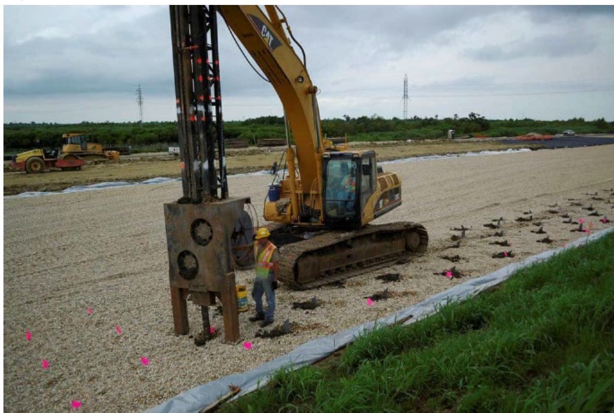
Figure 8-24: Example Wick Drain Installation
