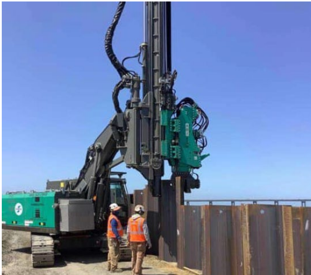
Figure 8-28: Example Pile Driving
