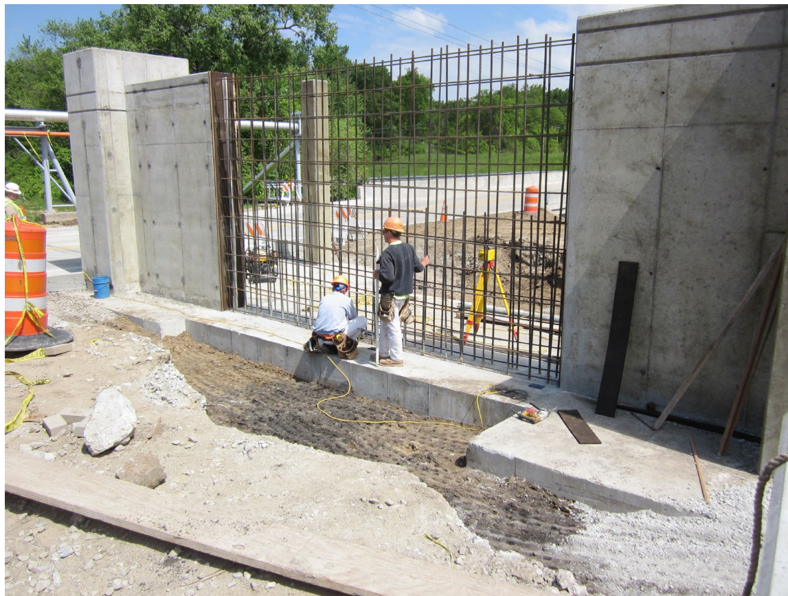
Figure 8-29: Example Closure Structure Construction
