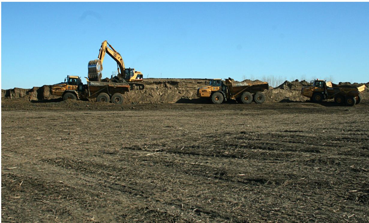
Figure 8-18: Example Borrow Source Excavation
