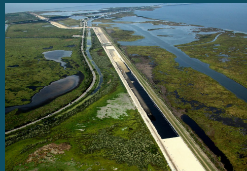
Levee removal in USACE's New Orleans District.
