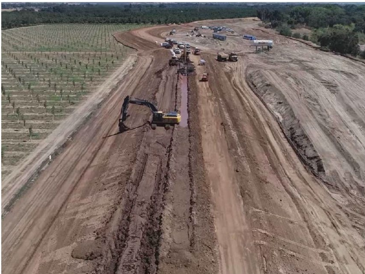
Figure 8-10: Aerial View of Levee Construction
