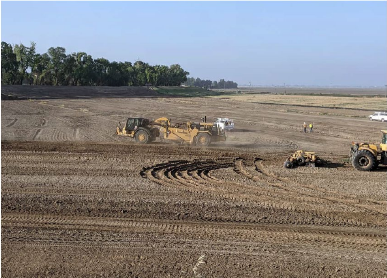
Figure 8-16: Example Levee Subgrade Preparation
