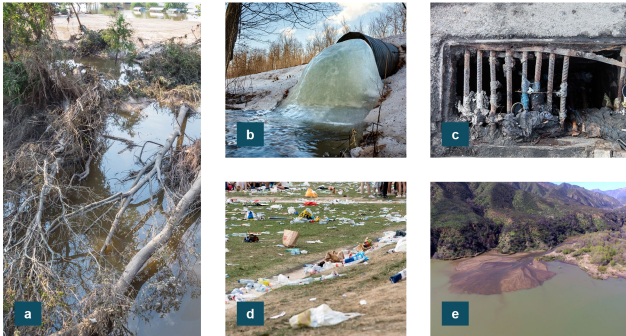
Figure 9-27: Examples of Vegetation and Debris Blocking Drainage
