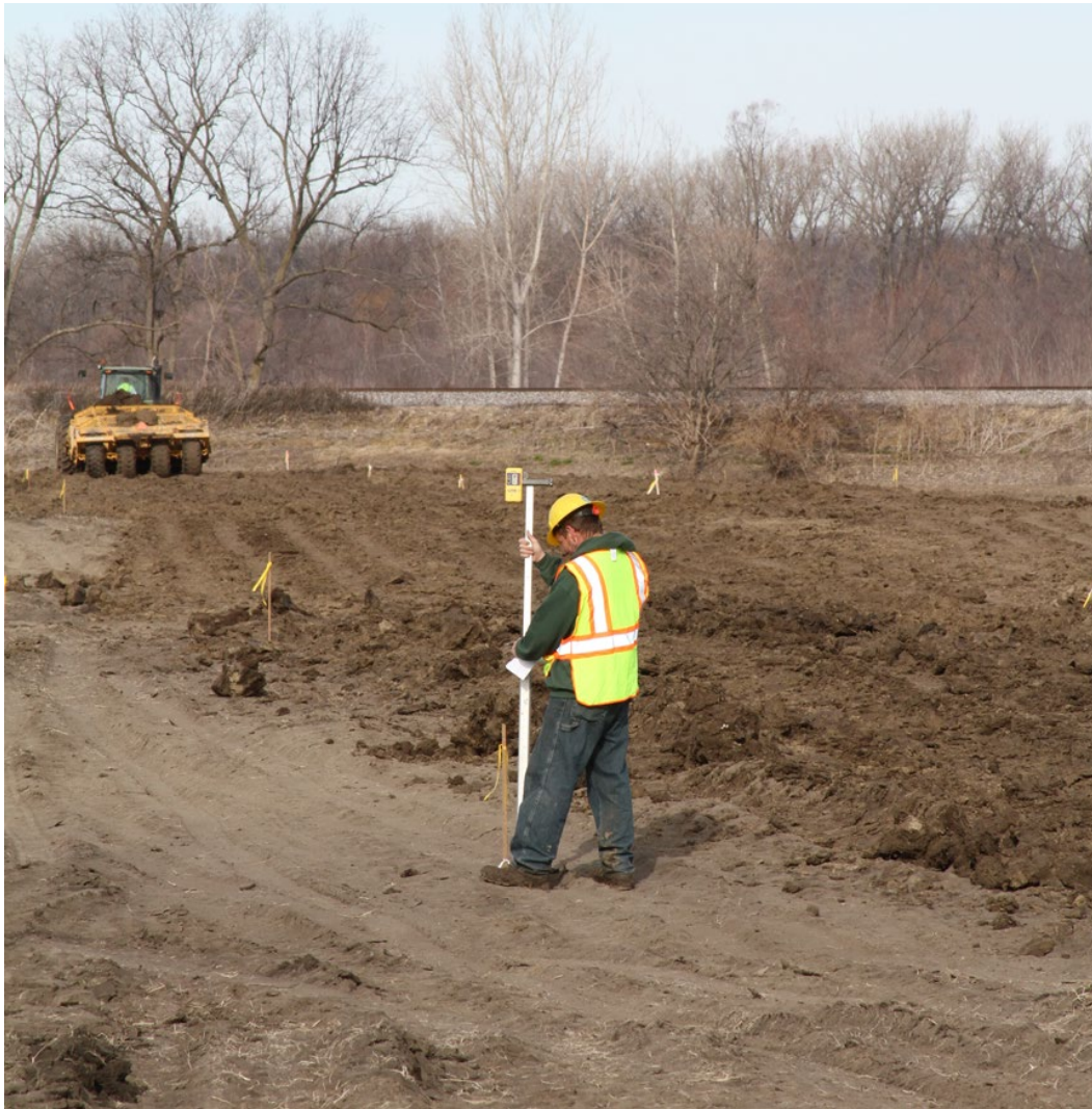
Figure 8-15: Example Survey Control
