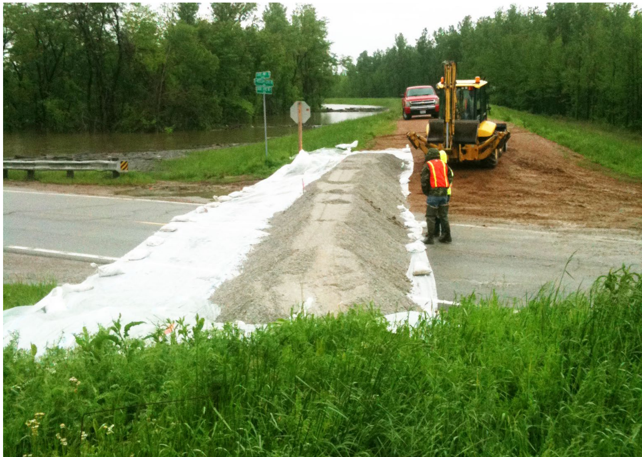
Figure 2-33: Example Earthen Fill with Plastic
