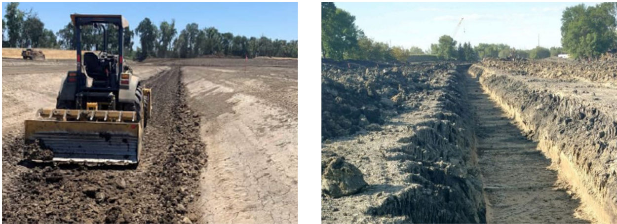
Figure 7-16: Example Inspection Trench
