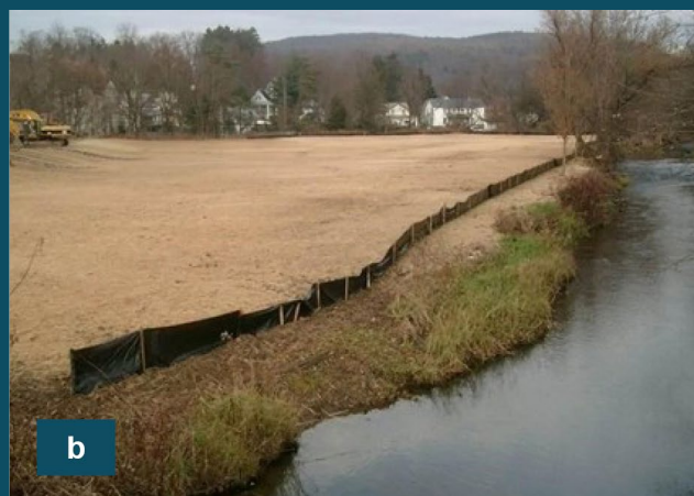
(a) The West Brook site before restoration. (b) The West Brook site after fill was removed and graded to the correct elevation and slope to allow water to spread out onto the floodplain.
