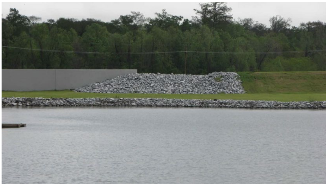
Figure 8-31: Example Levee Transition Connection (Embankment and Floodwall)
