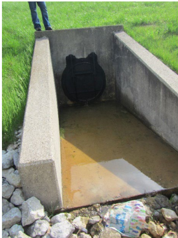
Figure 7-44: Example Headwalls with Flap Gates
