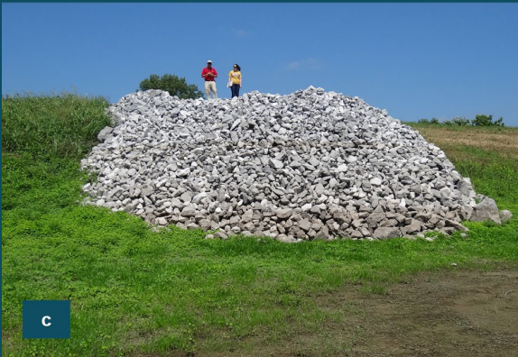
(a) Sinkhole caused by a buried pipe failure. (b and c) In 2013, emergency levee repairs occurred at a pipe failure along the Mississippi River. (d) A second pipe failure occurred a few years later at the same Mississippi River site.
