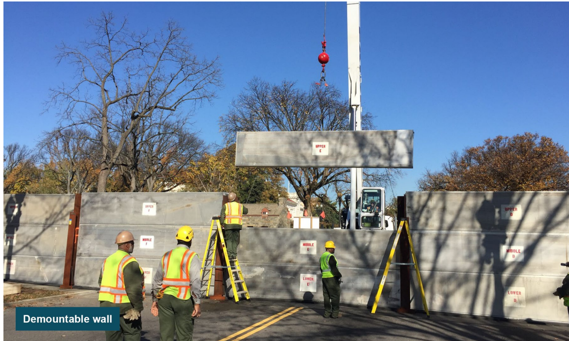
Figure 7-30: Example of Demountable Floodwall
