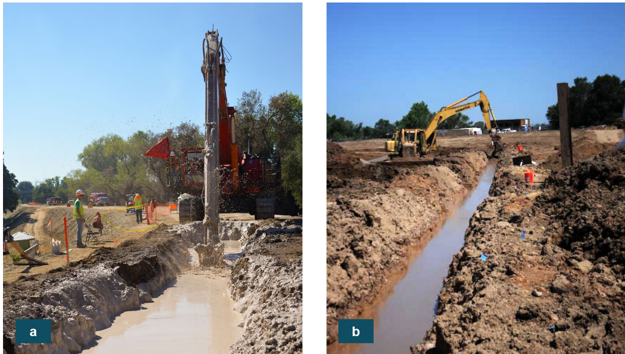
Figure 8-32: Example Open-Trench Cutoff Wall Construction
