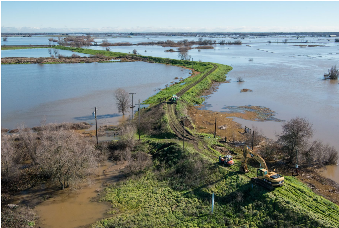
Figure 10-13: Workers Repair a Levee
