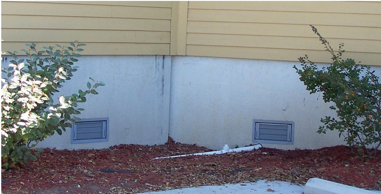
Figure 12-10: Wet Floodproofed Building with Flood Openings
