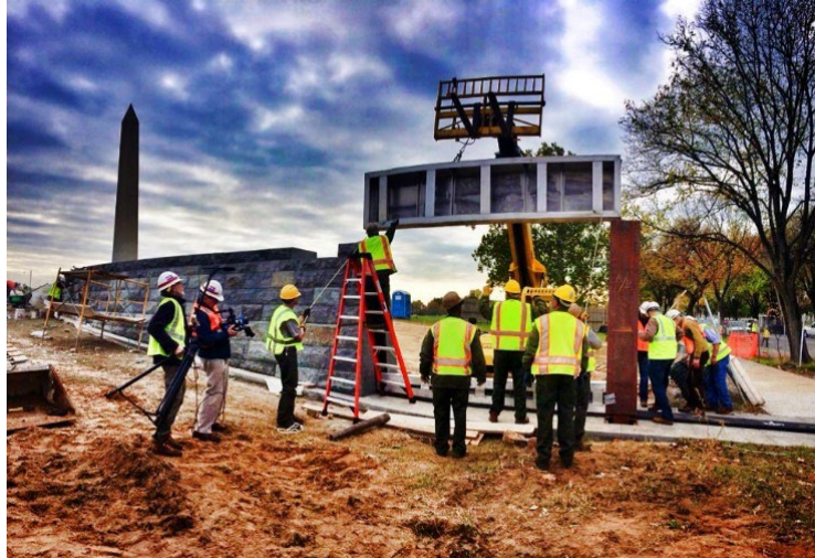
Test closure of the 17th Street levee in Washington, D.C., provides an opportunity to engage the public on the importance of the test and the benefits the flood risk reduction structure provides.
